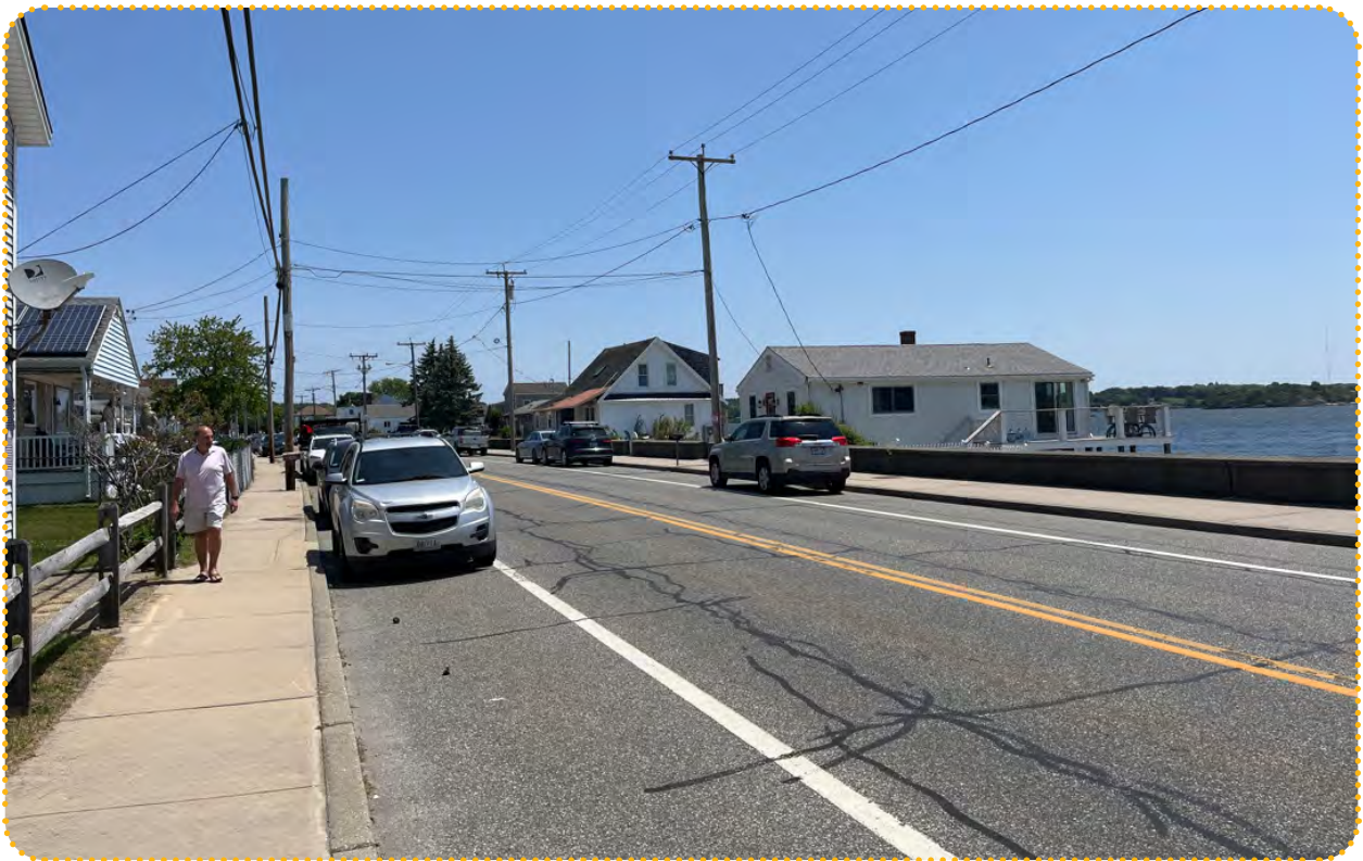
Existing conditions on Park Avenue
