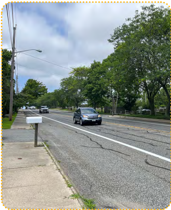
Existing conditions on Turnpike Avenue
