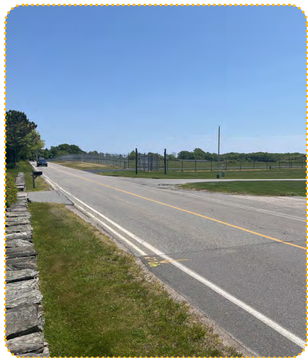
Existing conditions on Oliphant Lane
