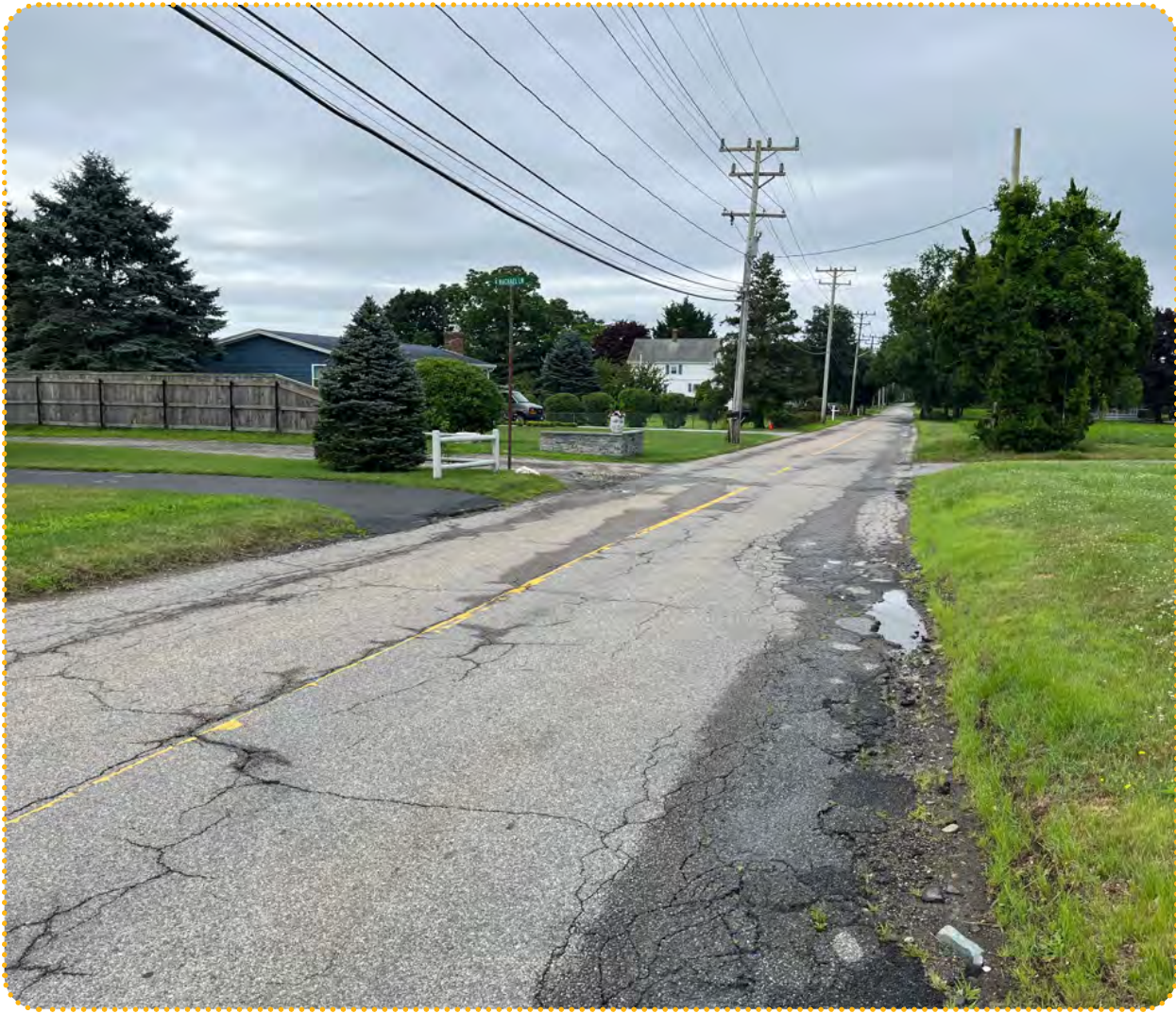
Existing conditions on Jepson Lane
