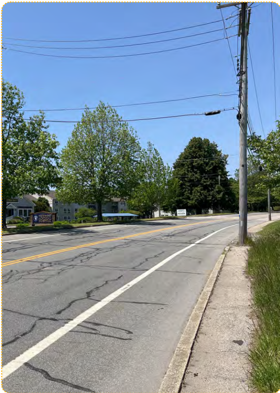
Existing conditions on Valley Road
